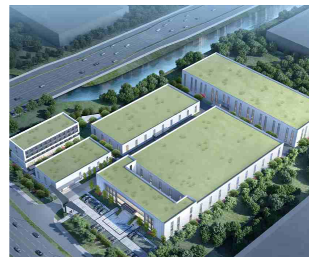
Phase II factory under construction
